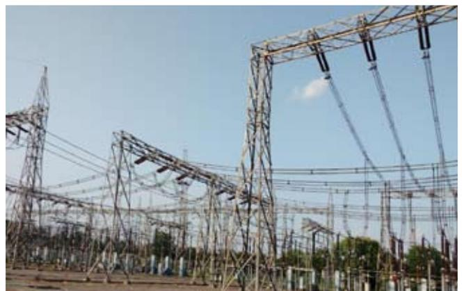
**Fig. 1 :** Air Insulated Substation with Gravel Surface
