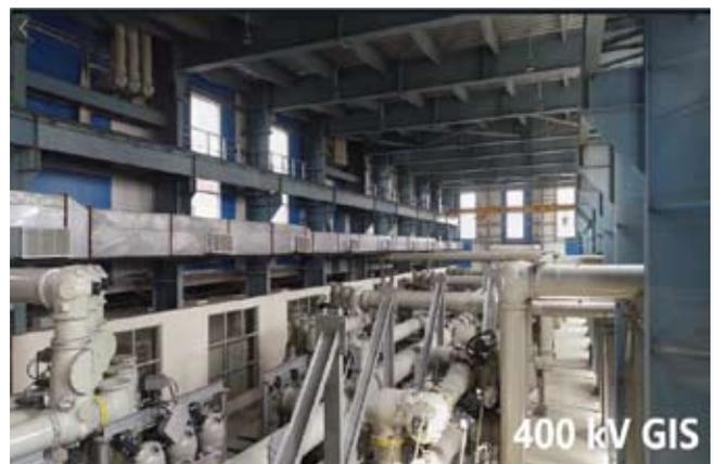
**Fig. 1 : 400 kV Gas Insulated Switchgear**
