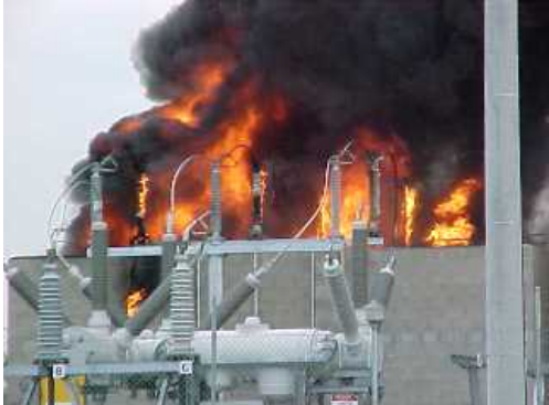
Ph 2. OIP bushing failure causes fire in transformer but fire contained by sound enclosure
