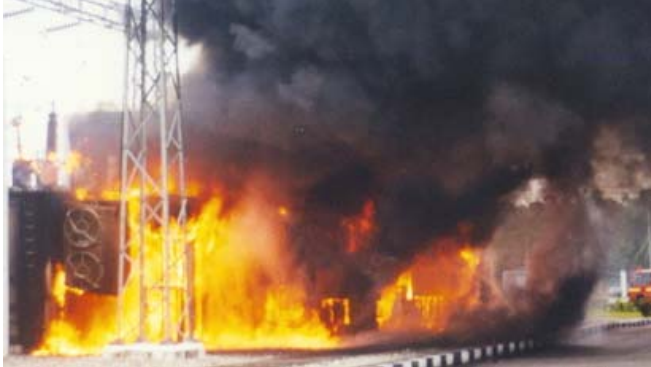
Ph 1. OIP bushing failure and oil spilling into common cable trench causes fire in two 90 MVA transformers
