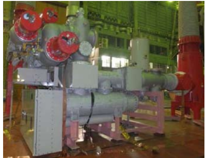
Fig. 7 : Prototype 420 kV GIS under dielectric test
